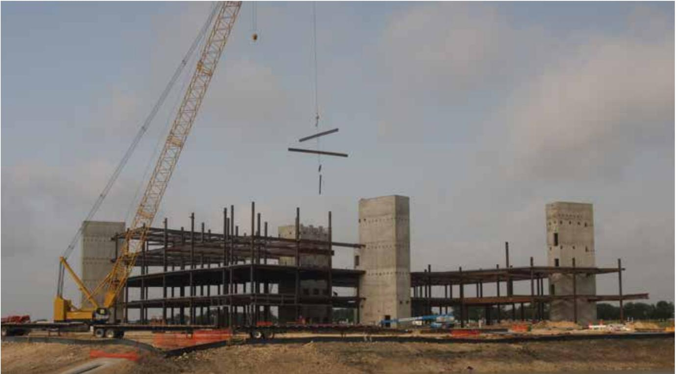
▲ Texas Health Harris Methodist Hospital Alliance, an IPD steel project, was detailed and fabricated by Alpha/SteelFab after they assisted in converting the design from the original concrete concept.
