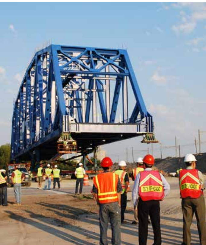
▲ Rolling in the 394-ft-long, 2,375-ton steel truss railroad bridge on SPMTs.
