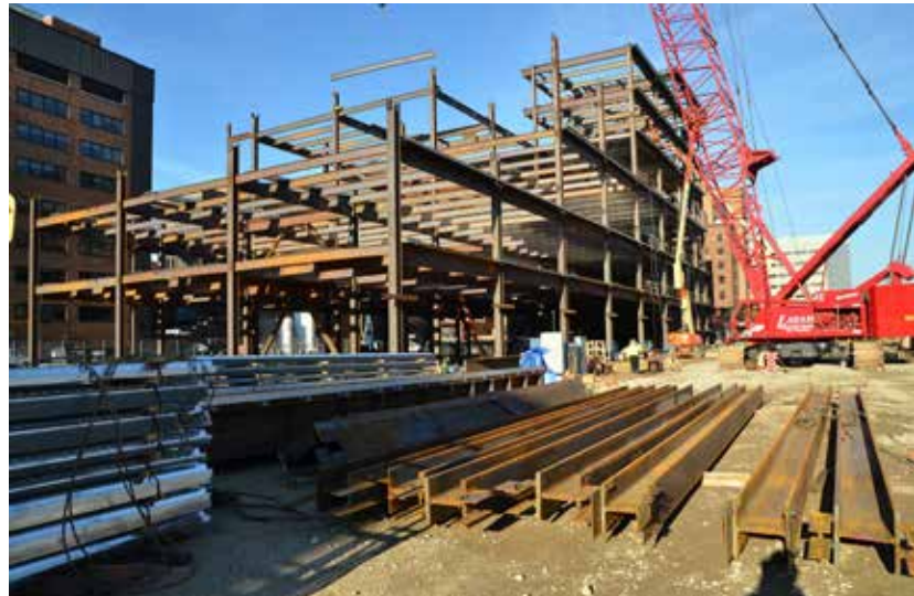
▼ The hospital, designed via a BIM approach, contains nearly 200,000 sq. ft of steel-framed space.
