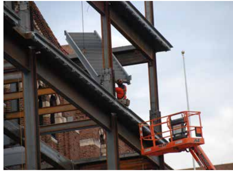
▲ Installing a staircase.
