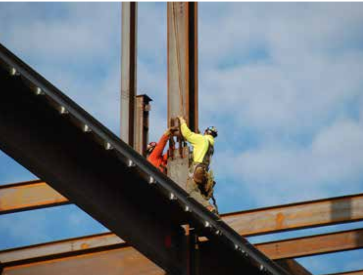
▼ Fitting up a column.
