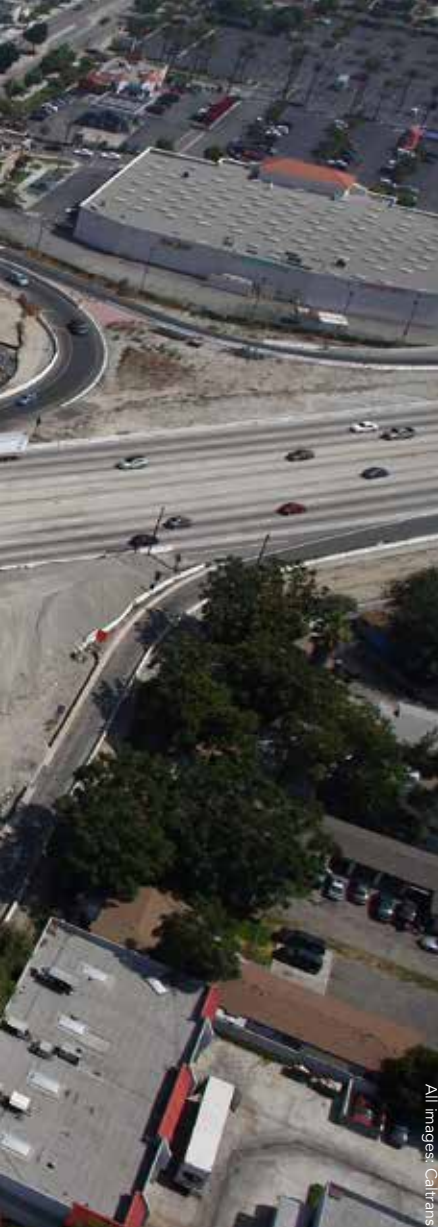
▲ The new Baldwin Park Overcrossing is a four-span steel I-girder bridge with a total structural length of 478 ft.
