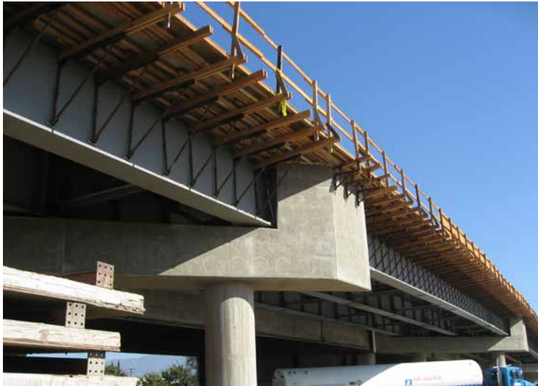
▲ The new Baldwin Park Overcrossing is a four-span steel I-girder bridge with a total structural length of 478 ft.
