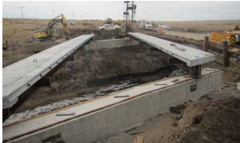
▲ Allied's first project using its Rapid Bridge System: the Maxwell Coulee Bridge, about 20 miles east of Jordan, Mont.
