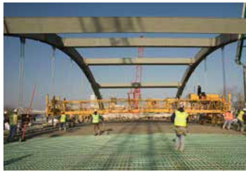
▲ Construction of the deck.
