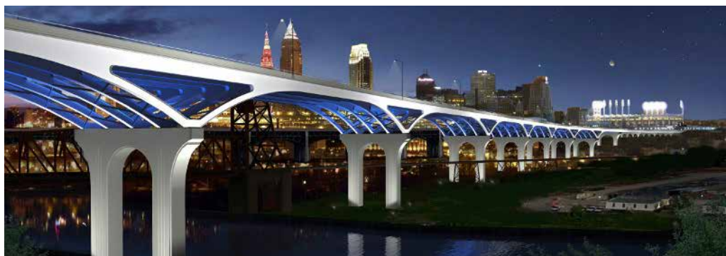
▲ The five-lane bridge will soar 120 ft over the Cuyahoga River at its highest point.
