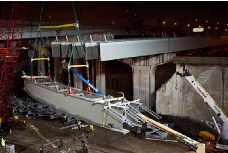
▲ The westbound bridge will use 20,000 tons of structural steel in all.
