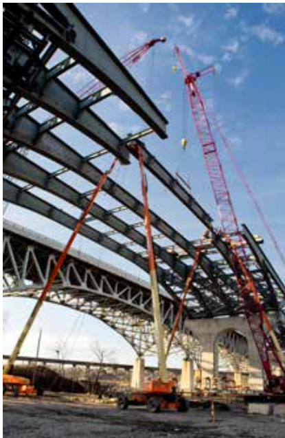
▲ The new westbound portion of the Innerbelt Bridge under construction next to the existing 1959 bridge.
