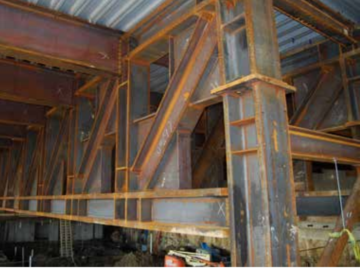
◀ 10-ft-tall trusses in the practice facility.
