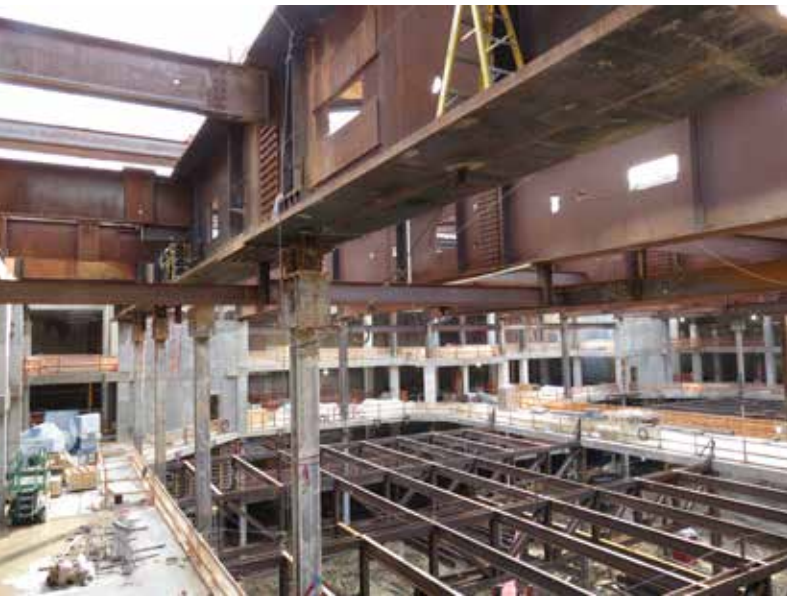
◀ Steel plate girder and grand ballroom steel truss floor framing.
