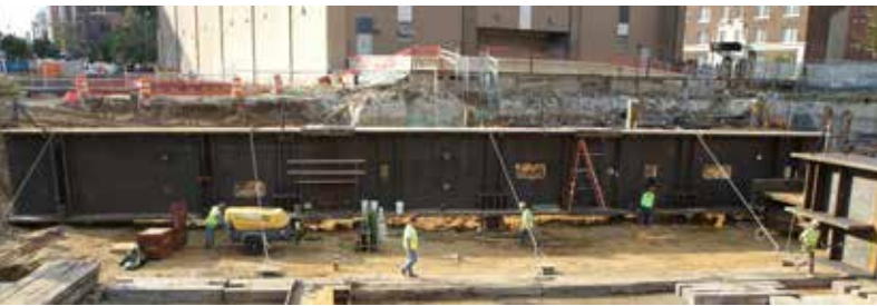
◀ Erection of the first plate girder prior to the beginning of top-down construction.
