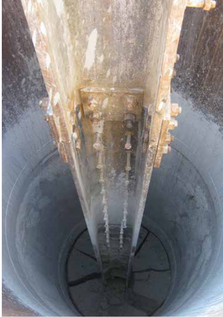
▲ Typical below-grade top-down steel column.
