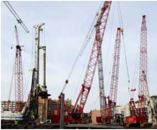
◀ The congested site in the middle of D.C. included tower cranes, drilled shaft rigs, excavation rigs and crawler cranes.
