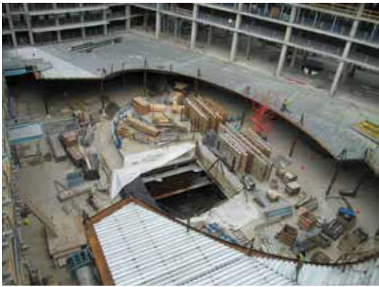
◀ Looking down into the ground-floor atrium.
