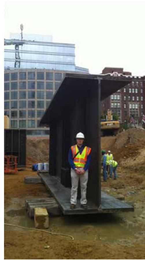
◀ Steel plate girder and grand ballroom steel truss floor framing.
