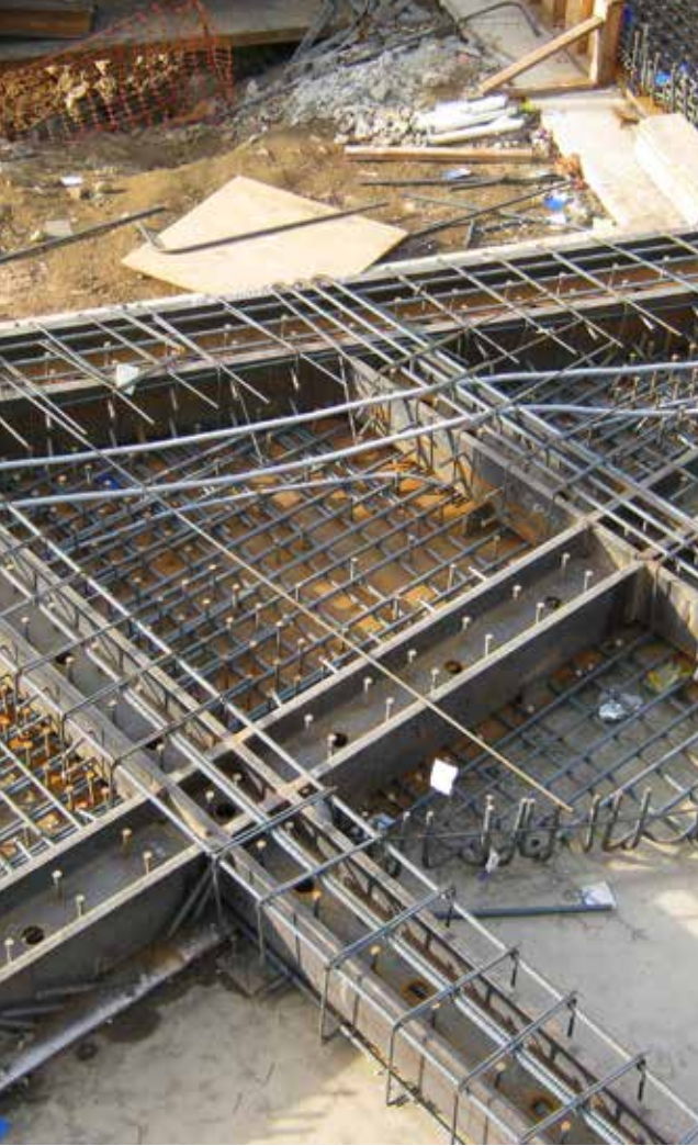
▲ Wide-flange and plate steel slab reinforcement.
