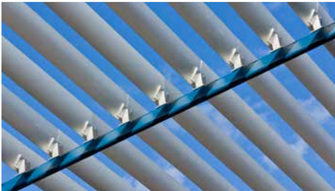
▲ The northern side of the canopy has a large, louvered trellis that allows abundant daylighting for the planting below.
