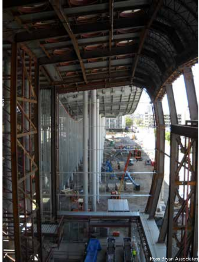
▲ A slightly different angle from left photo, with the 120-ft-tall, 36-in.-diameter columns in the background.
