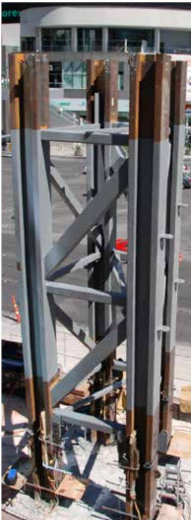
There are nine individual LED cabinets, most of which (excluding the lower pole covers) were 65 ft long by 16 ft, 9 in. wide by 10 ft tall. The heaviest was the top cabinet, at 23.5 tons, and the roofing provides drainage through the sign as well as davits that give access to the exterior of the sign for periodic washing of the faces. Most of the electrical components can be maintained from the inside, with each cabinet level having 750 sq. ft of interior floor space.
