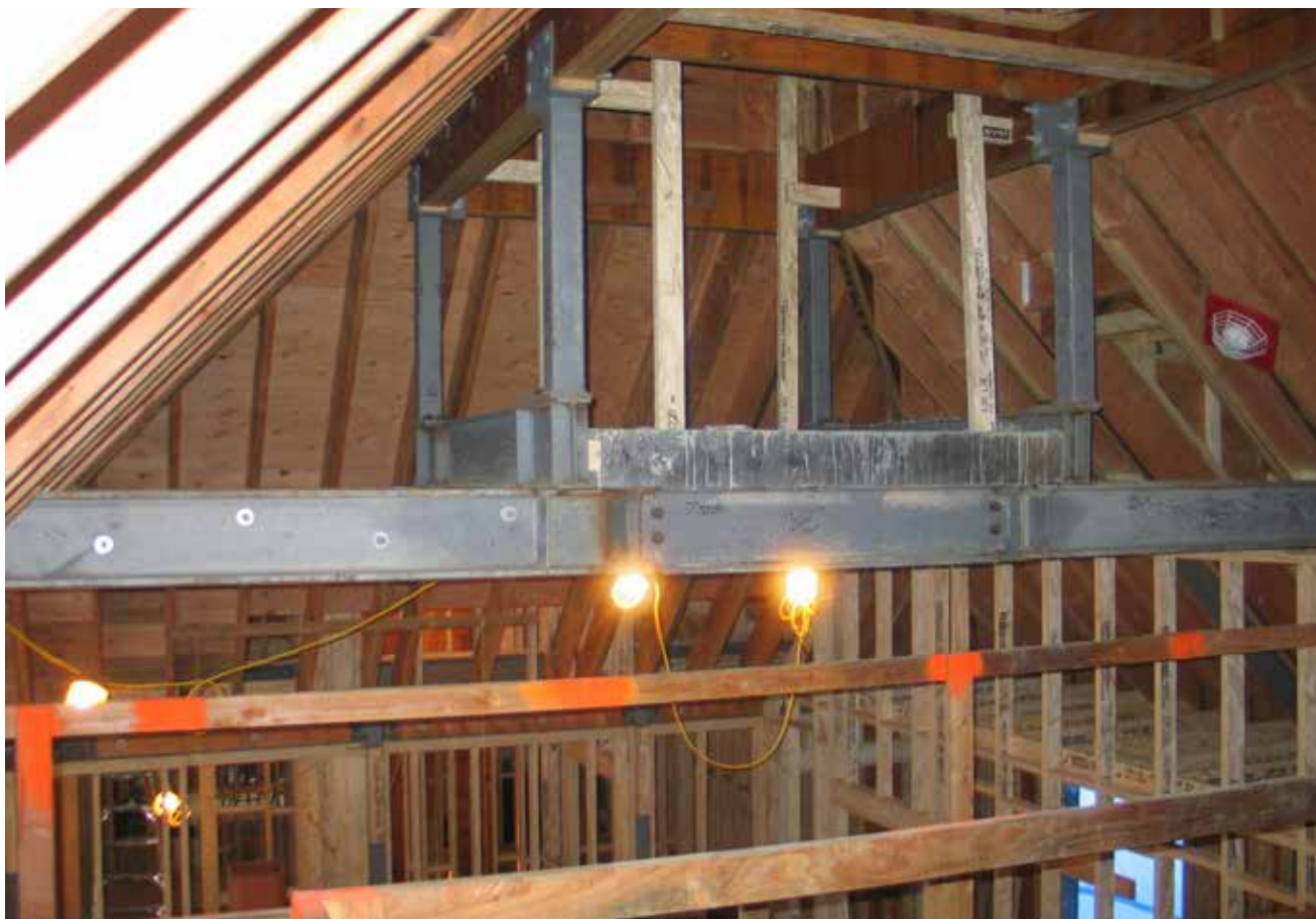
◀ The steel framing system for the pool house.
