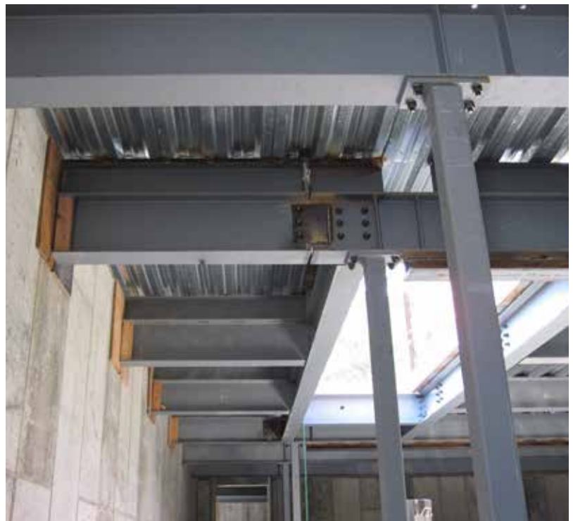
▼ Garage floor composite steel construction.
