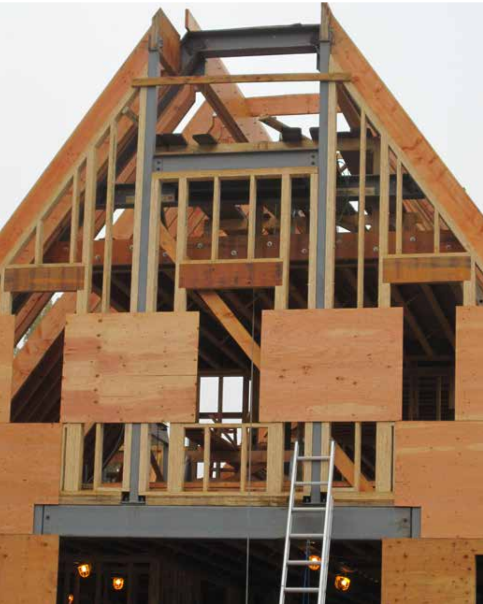
◀ Steel transfer system at a gable end of the building.
