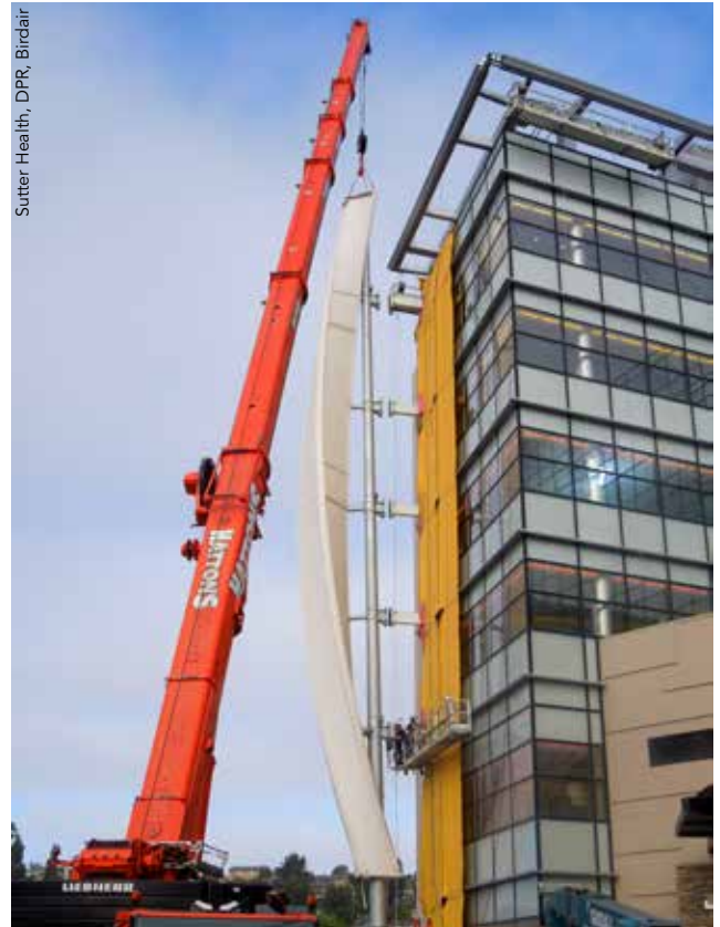
◀ ▲ Diagrammatic view and installation of the signature 125-ft-tall spire element.
