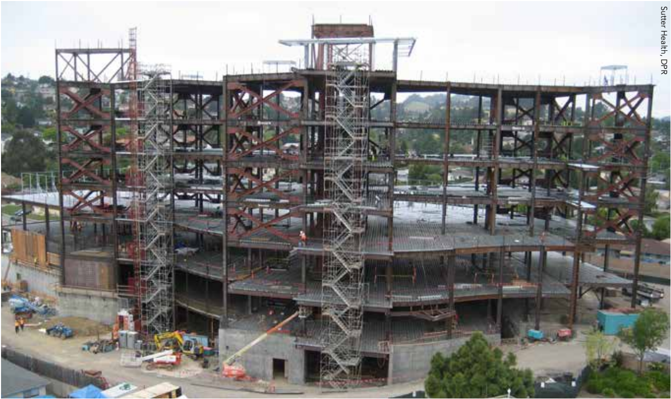
▲ Construction after main steel erection.
