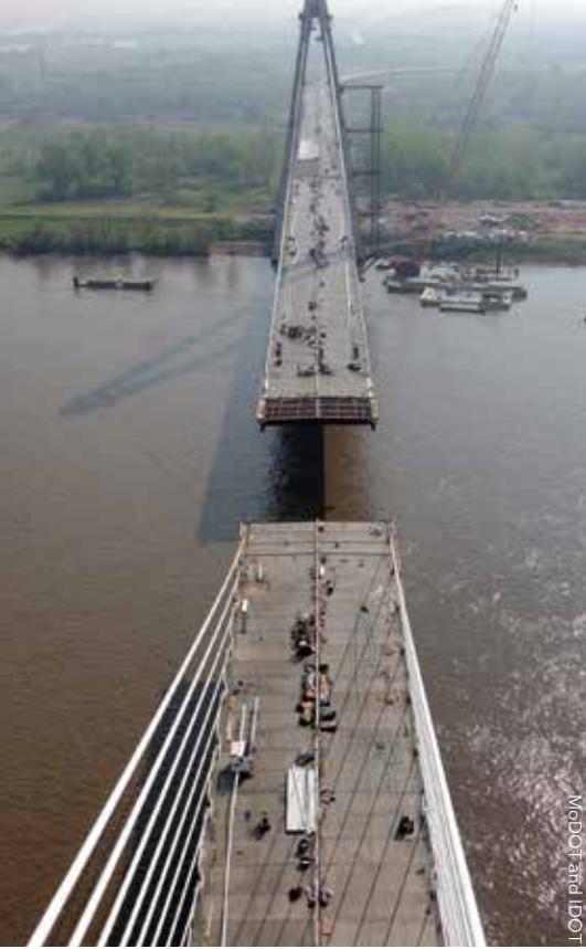
▲ The Illinois and Missouri sections, before being joined in the middle.
