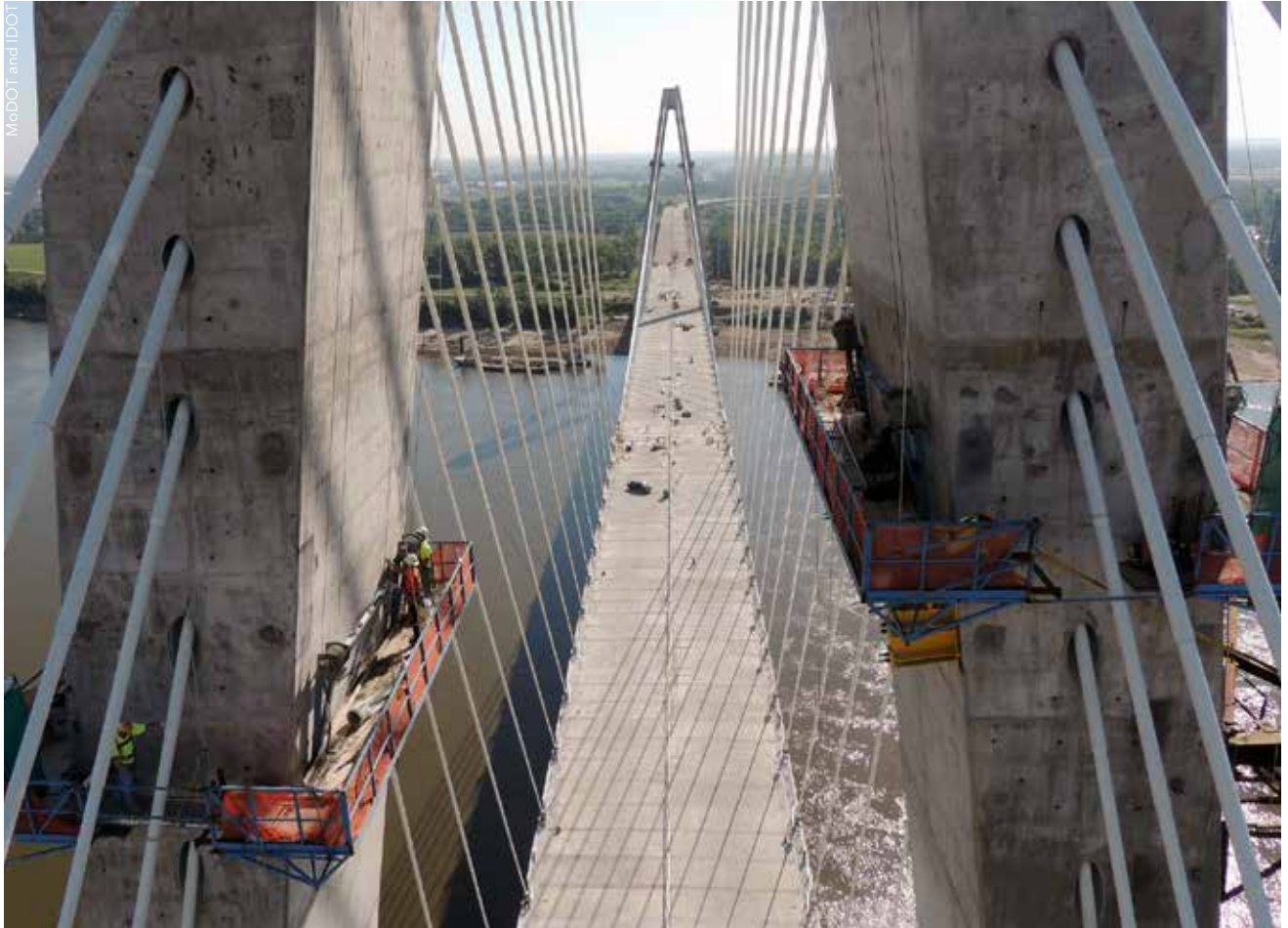
▲ A view from one of the 400-ft-tall pylons, with the Illinois and Missouri sections connected.
