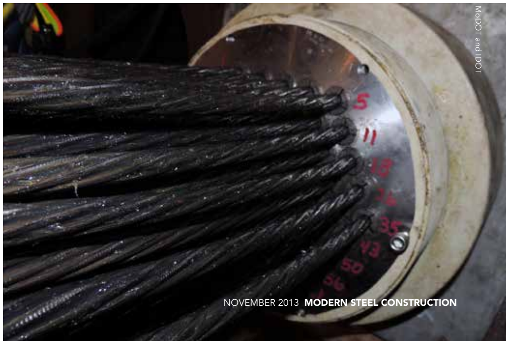
▼ A cable anchorage.
