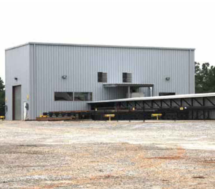
▼ The 2,800-sq.-ft material processing building.
