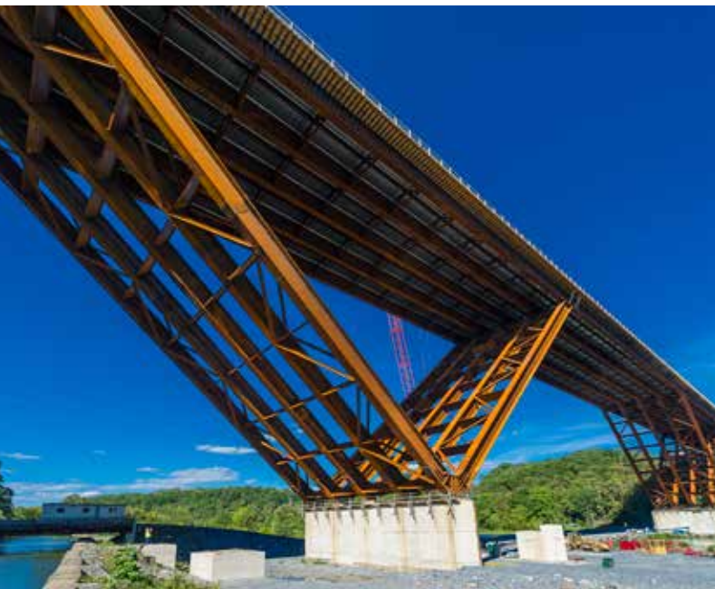
▲ The four-lane bridge is part of a new alignment for WV9, which formerly accessed the valley via a winding, two-lane road.
