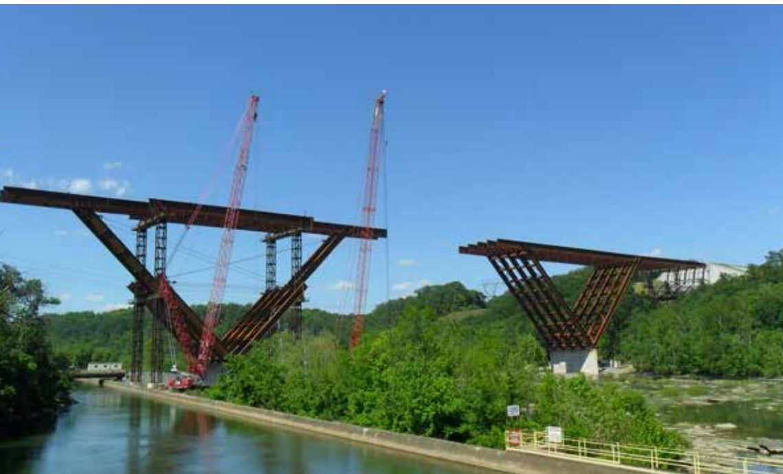
▲ The superstructure consists of a five-girder, four-substringer system supported by five lines of delta legs—one for each girder.
