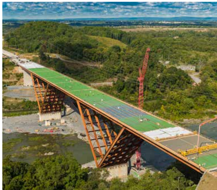
▲ The structure was modeled in 77 stages, each defined as the amount of work that could be completed during a shift or between any appreciable wind or thermal event.
