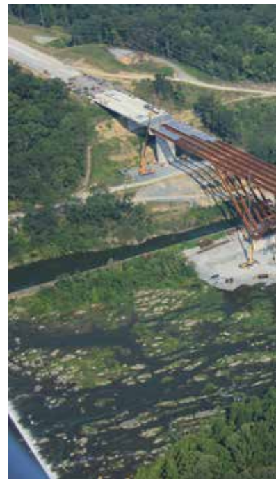
▲ The superstructure consists of a five-girder, four-substringer system supported by five lines of delta legs—one for each girder.
