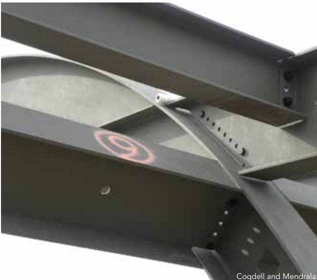
▲ Shop-fabricated utility penetrations in the steel framing.
