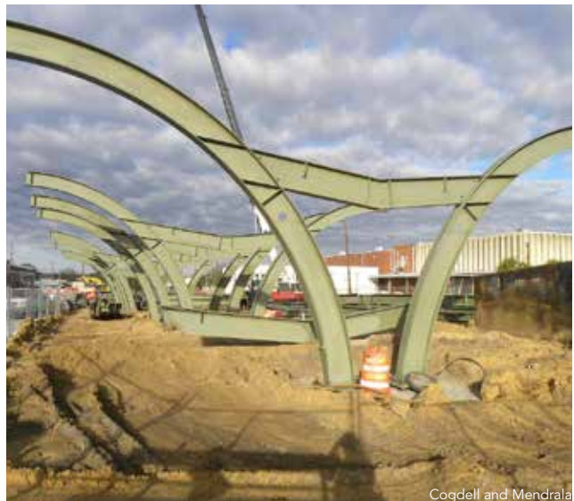
▲ The transfer canopy during erection.
