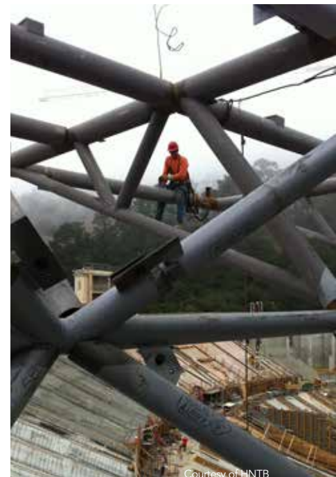
▲ Working on the HSS of the cantilevered balcony.
