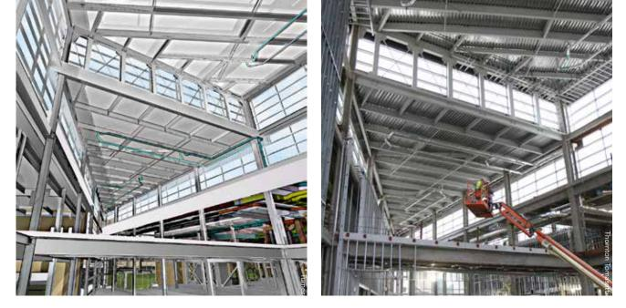
The truss diagonals consisted of double 1¼-in. tension rods in one direction and single 1¾-in. tension rods in the opposite direction. Steel wide-flange columns surrounding the high bay space support a grid of HSS girts that provide lateral support to the glass curtain wall.
