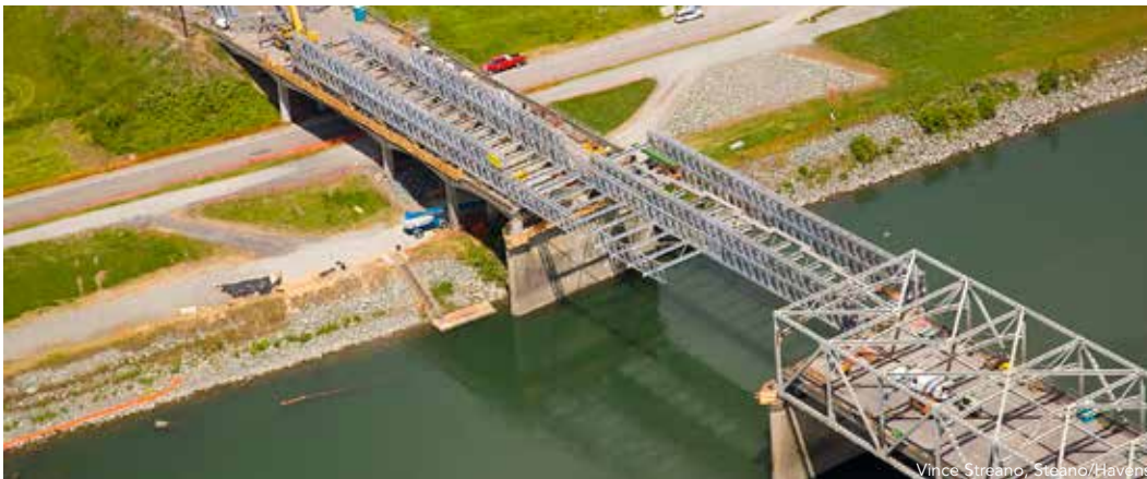
◀ Erection of the temporary spans.
