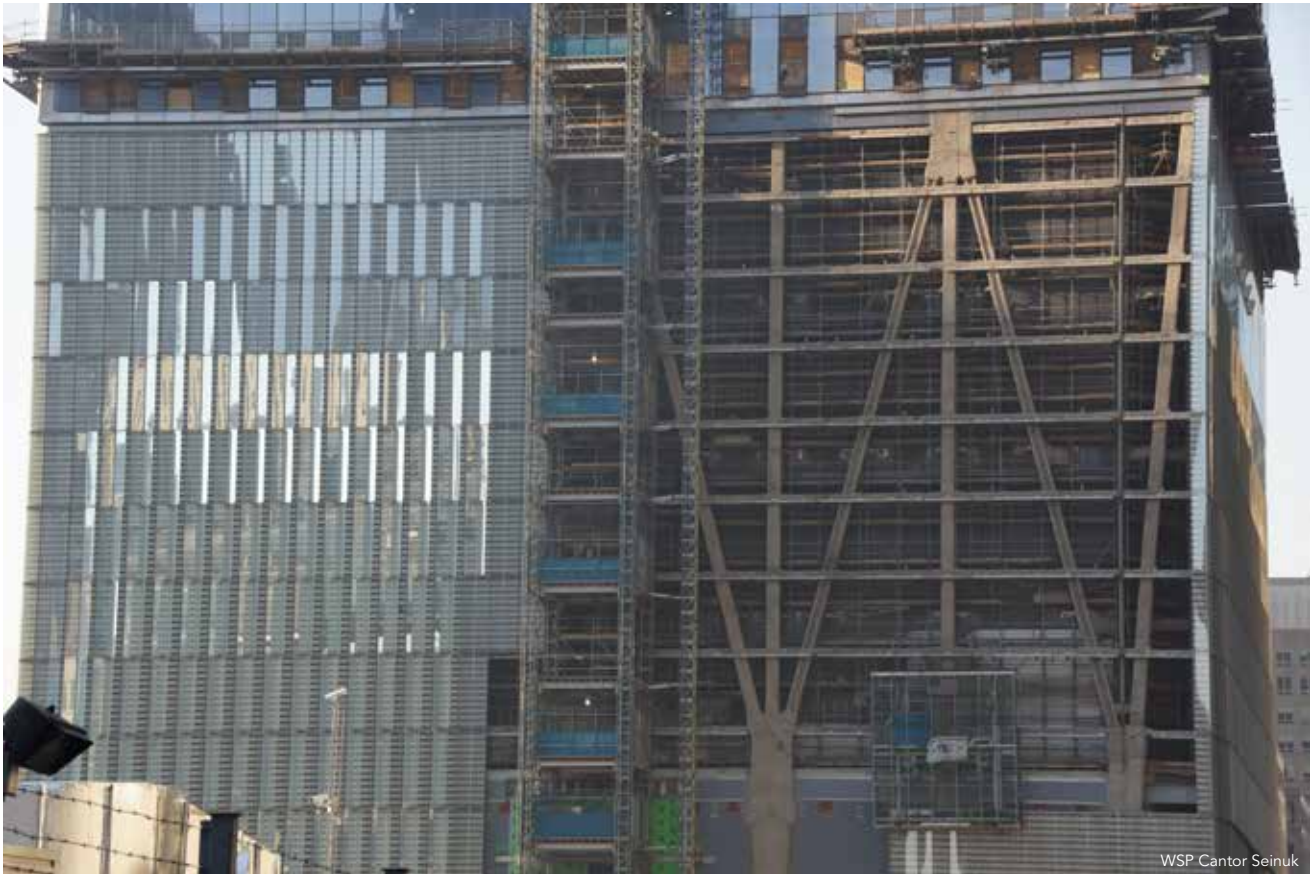
▲ The structural system at the base of the tower.
