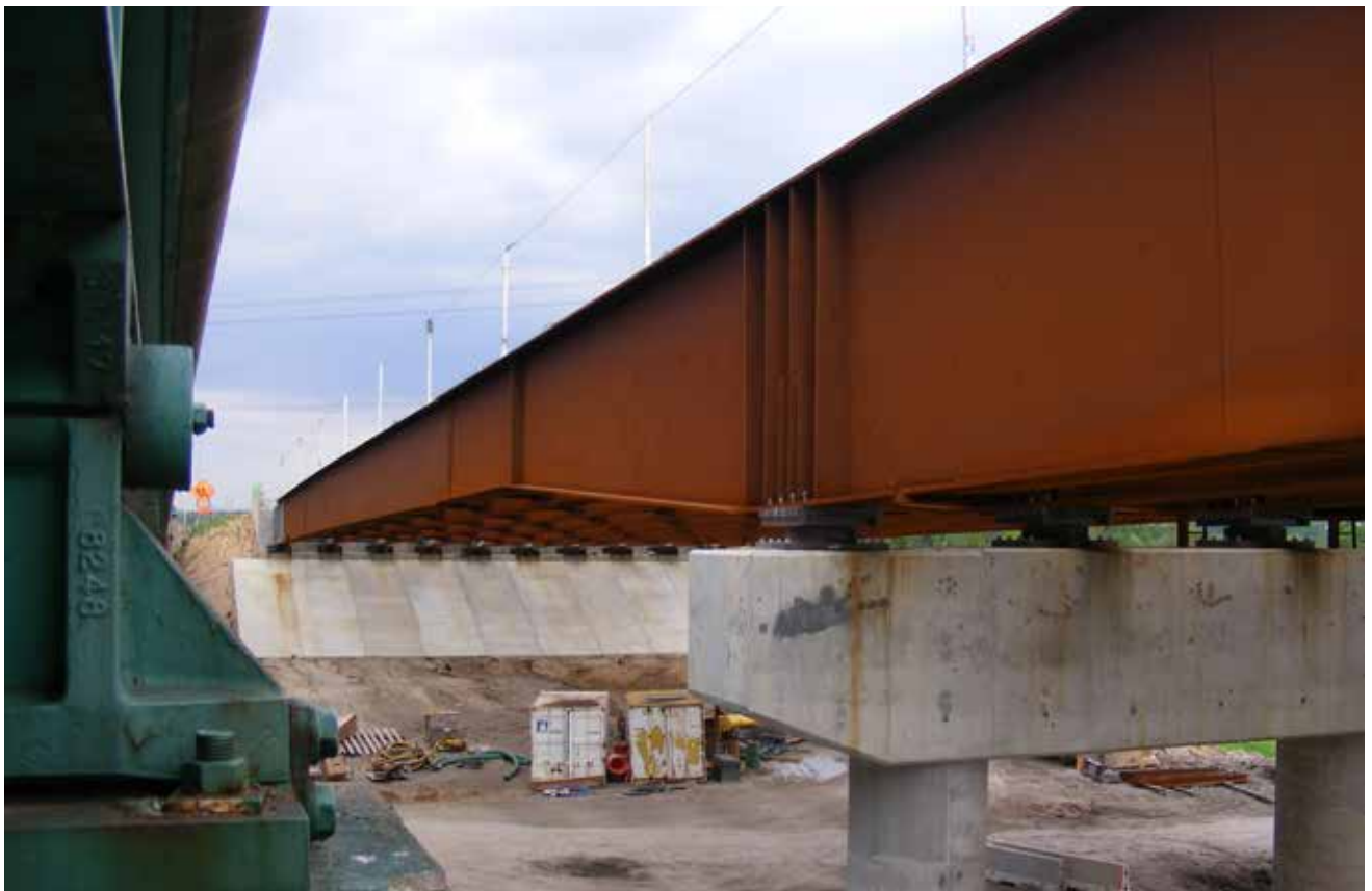
▼ Girder web depth transition at Pier 1 of the I-270 bridge.
