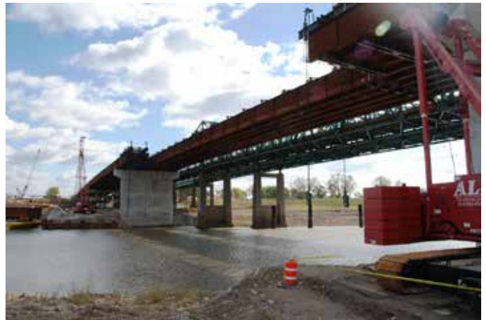
▲ The steel superstructure of I-270 before the last lift.
