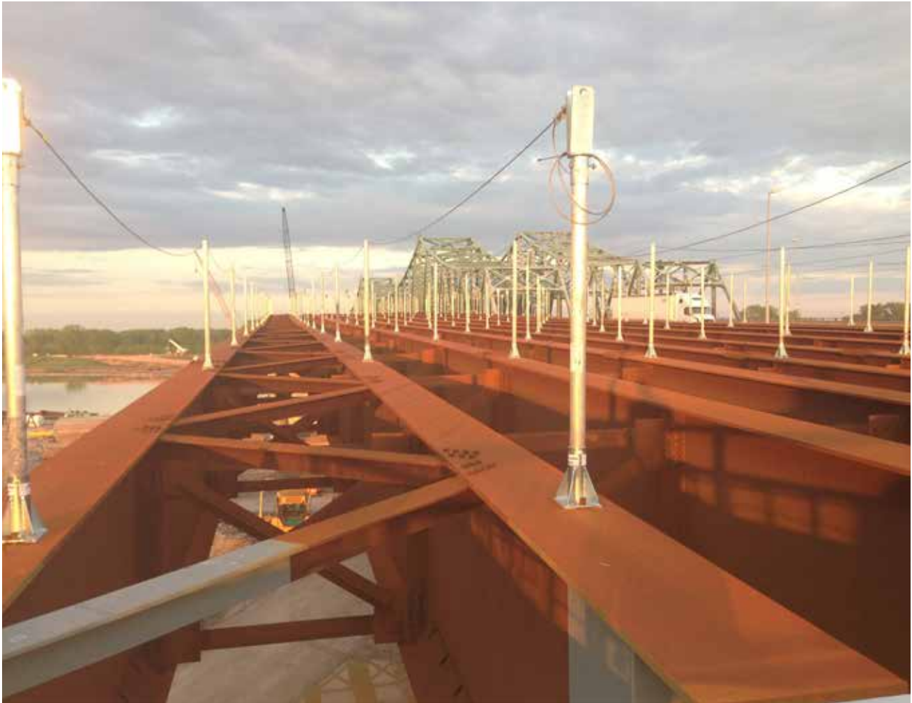
▲ Top flange lateral bracing for the bridge.
