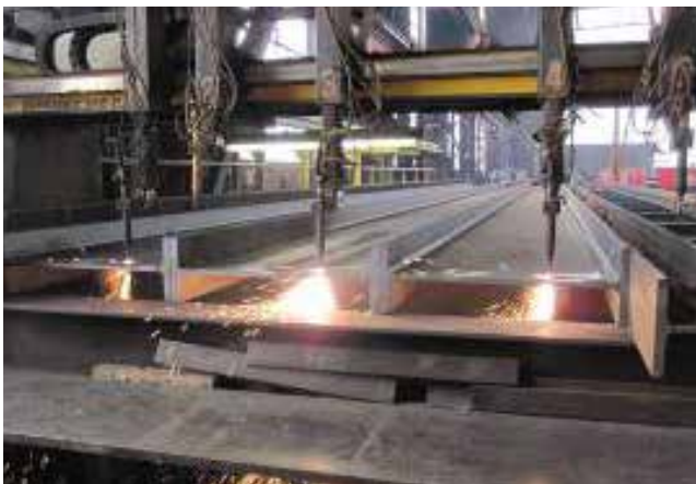
▼ Steel fabrication of the Pöcking Bridge.
