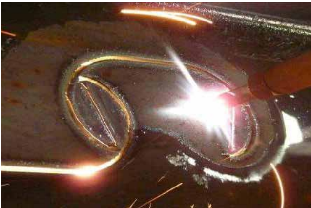
▲ The cutting pattern of the MCL composite dowel.
