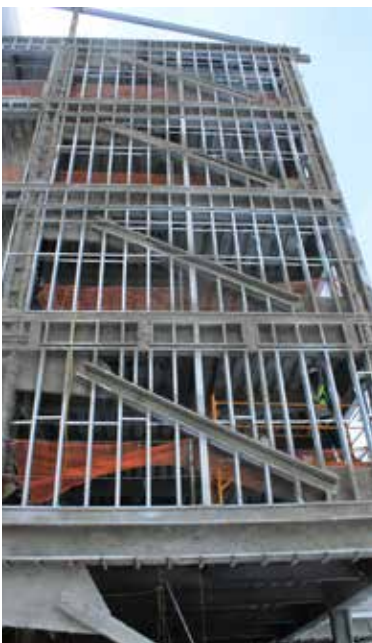
▲ BRBs abound in the Adult Behavioral Health Center. ▼ Diagonal bracing in one of the residential buildings.
