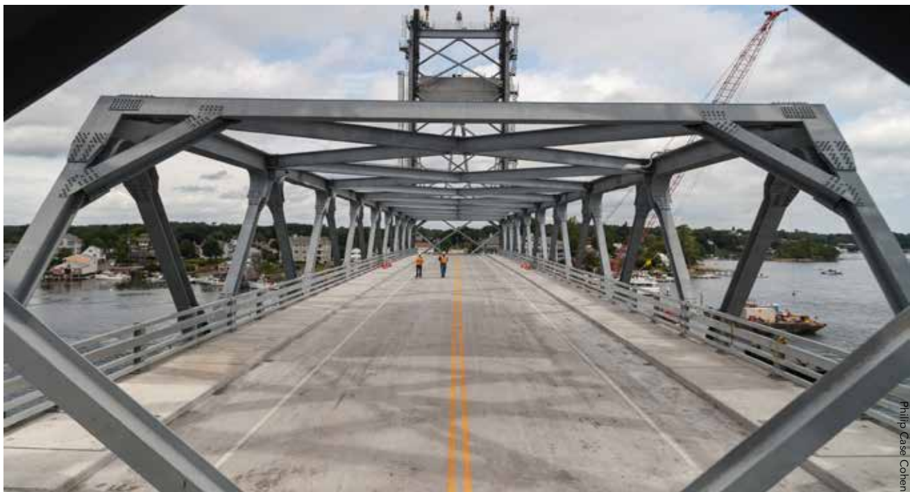
▲ The design features two 11-ft through lanes, two 5-ft shoulders for bicyclists, two 6-ft sidewalks and overlooks at both flanking spans.
