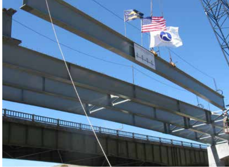
▲ Setting the middle section of the last girder.
