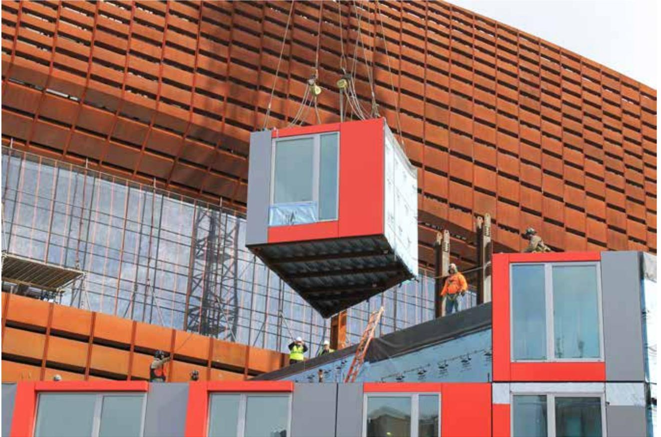
**WITH BARCLAYS CENTER** (home of the NBA's Brooklyn Nets) looming in the background, a high-rise residential project is coming together—block by block. When it's completed next year, B2 will be the tallest modular building in the world. The 32-story tower is one of more than a dozen structures planned for the 22-acre Atlantic Yards site in Brooklyn. The structure's 4,000 sq. ft of retail space and
