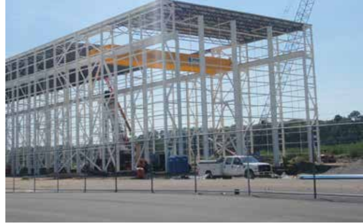
▶ ▲ The manufacturing building required clear heights of over 70 ft and clear spans of up to 90 ft.
