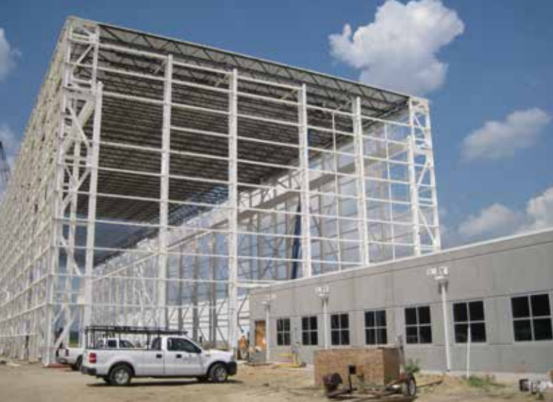
▶ ▲ The manufacturing building required clear heights of over 70 ft and clear spans of up to 90 ft.
