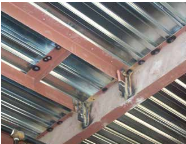
▲ A traditional welded roof penetration system.
