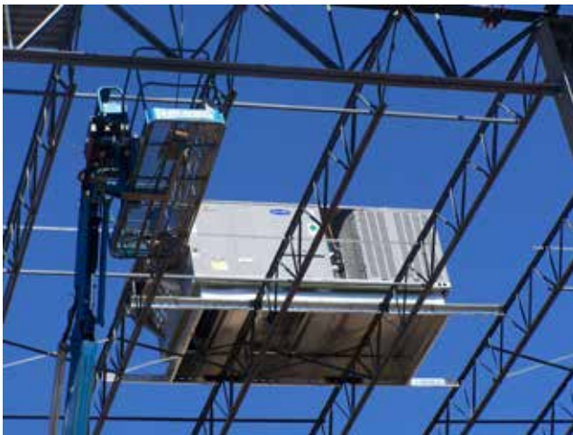
▲ A QuickFrame roof penetration before deck installation...
