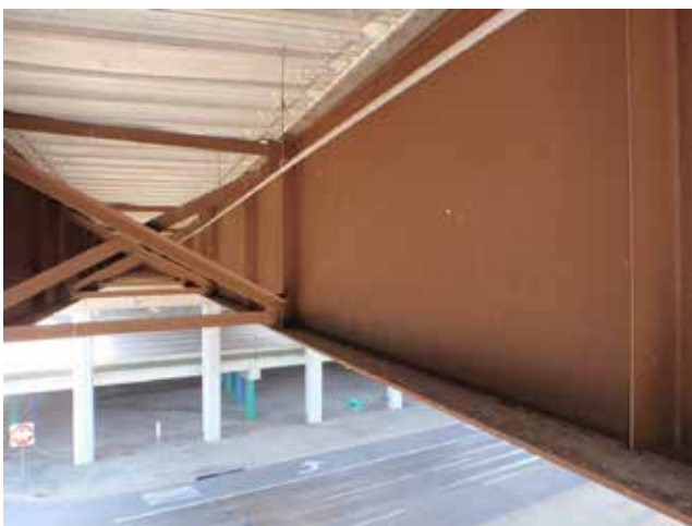
◀ Favorable performance of a UWS overpass.
