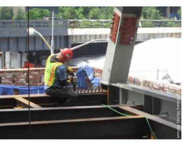
New steel at the upper levels frames into the preserved existing façade at the lower levels.
