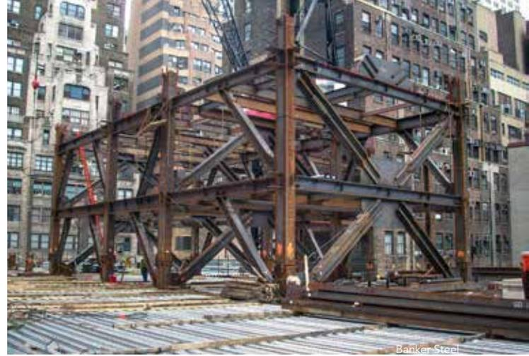
◀ ▲ Rooftop steel, including a stiff braced frame system around the central elevator core.
