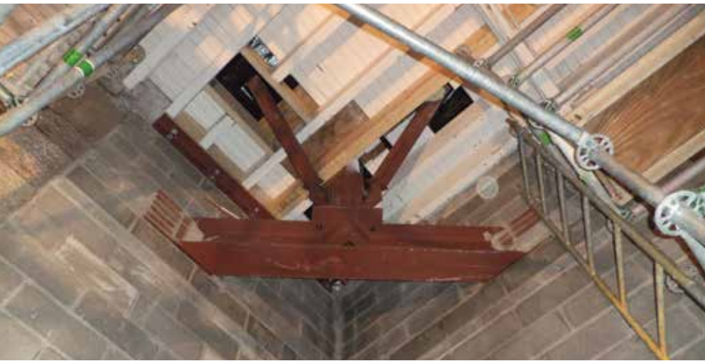
◀ Internal reinforcements within the reconstructed clock tower.
