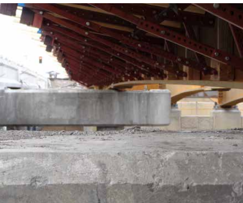
▲ Mechanically stabilized earth (MSE) walls were constructed in front of the abutments in order to minimize the span lengths, yet still provide for future Interstate widening. ◀ Steel superstructure connecting to the piers.
