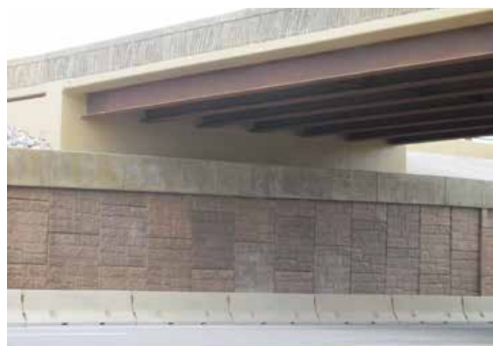
▲ Mechanically stabilized earth (MSE) walls were constructed in front of the abutments in order to minimize the span lengths, yet still provide for future Interstate widening. ◀ Steel superstructure connecting to the piers.
