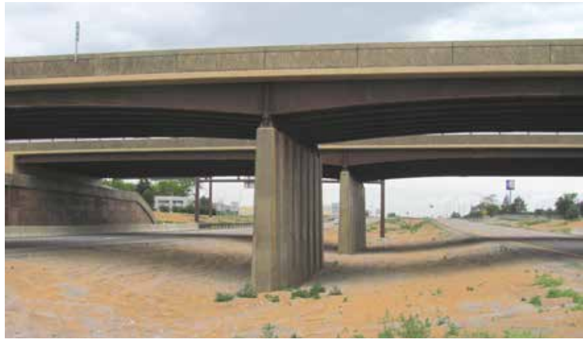
▲ To accommodate widening, corrugated metal pipe (CMP) sleeves were used in the MSE fills to prevent damaging the soil reinforcement when future piles are driven. The integral abutments eliminated the need for expansion joints and bearings at the ends of the girders. ▼
