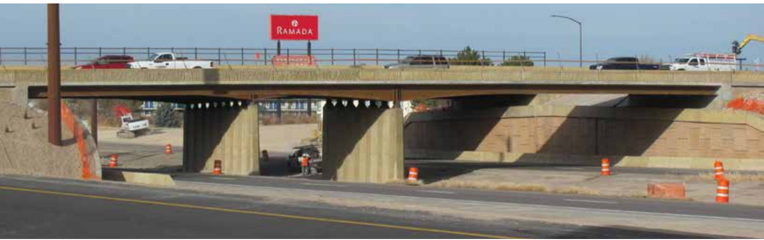
▲ To accommodate widening, corrugated metal pipe (CMP) sleeves were used in the MSE fills to prevent damaging the soil reinforcement when future piles are driven. The integral abutments eliminated the need for expansion joints and bearings at the ends of the girders. ▼
