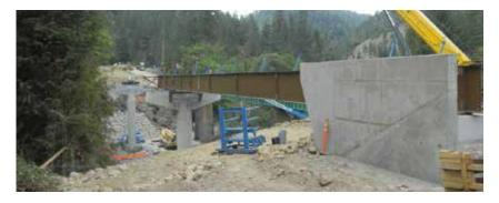
The new width is 31 ft, 4 in., providing a clear roadway width of 28 ft. Bridge abutments were founded on 2-ft, 6-in. drilled shafts socketed into bedrock.
