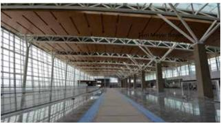
The airport trusses with cladding and skylight built above each; the bottom chord looks continuous because of the two A hidden bolted splice connections covered with a steel sleeve.
