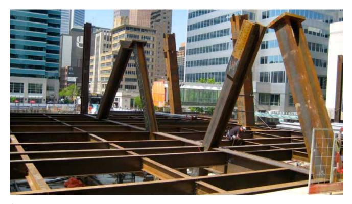
Installation of a two-story-tall transfer truss at the ground level of a 50-story office building; the truss transfers the loads of two 48-story-tall columns.
