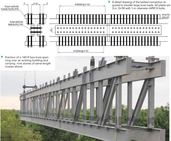
connections. However, when handling large trusses with large loads it is often impractical, even impossible, to transfer the loads through a bolted connection, so field-welded connections must be used. Field welded splices should be avoided as much as possible, especially when the connection is difficult to reach.
