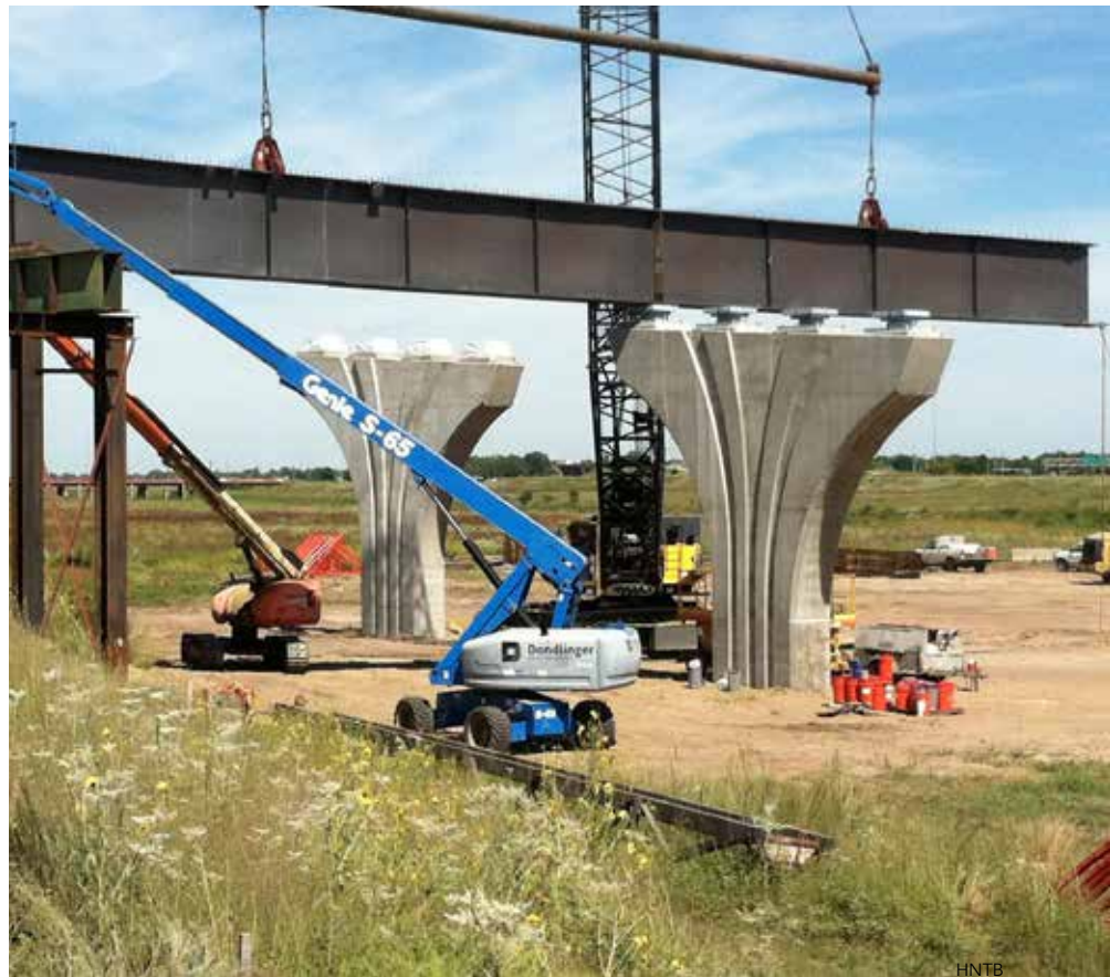
▲ Weathering steel was chosen to minimize future maintenance requirements.
