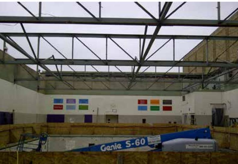
◀ Roof trusses for the original pool. Some members were reinforced while others were replaced.
