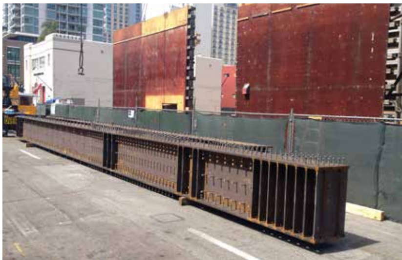
▲ A pair of transfer girders waiting to be lifted into place.
