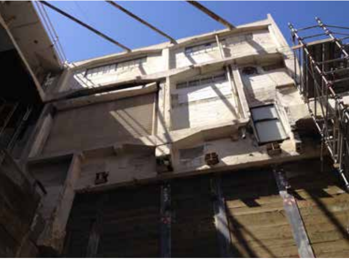
◀ The façade of the adjacent historic building, supported by stub beams off of soldier piles.
