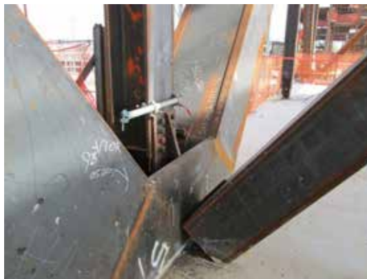
▲ The design team chose to form built-up nodes by using cheek plates aligned with the face-to-view in elevation plates of the box members. All axial loads, out-of-plane bending and in-plane shear were taken through the interface of the box member plates and cheek plates.
