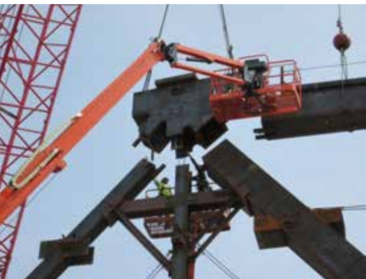
▲ The design team chose to form built-up nodes by using cheek plates aligned with the face-to-view in elevation plates of the box members. All axial loads, out-of-plane bending and in-plane shear were taken through the interface of the box member plates and cheek plates.
