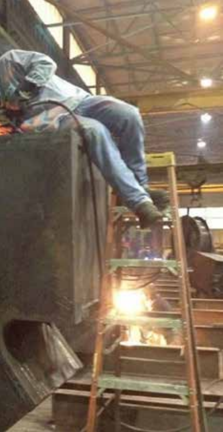
◀ Fabricating the nodal connections.
