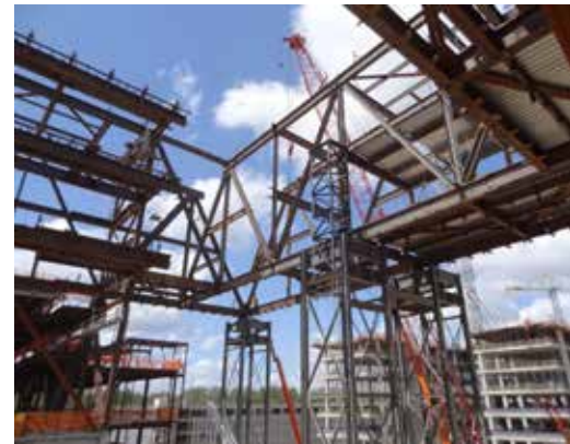
▲ To facilitate erection concerns, the Cube was built on top of temporary jacking assemblies, and permanently resting the Cube on the pot bearings occurred after substantial completion of its erection.
