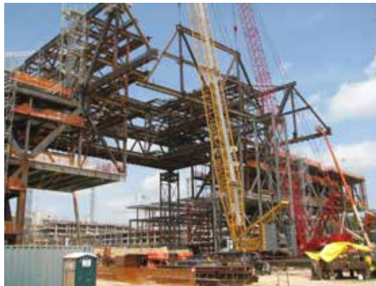
▲ To facilitate erection concerns, the Cube was built on top of temporary jacking assemblies, and permanently resting the Cube on the pot bearings occurred after substantial completion of its erection.
