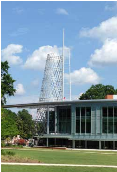
▲ The first ring measures just over 19 ft in height, rings two through seven measure 13 ft and the eighth ring is 5 ft. Each ring section comprises separate erectable panels of four sweeps and one counter-sweep.
