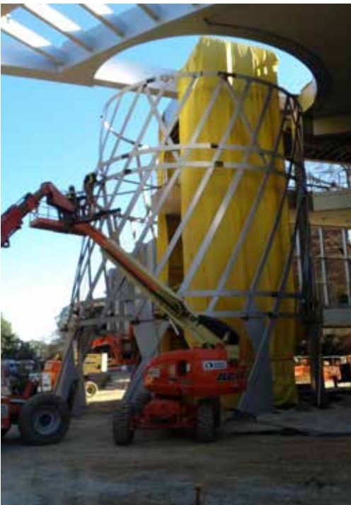
▲ The total number of rolled sweep and counter-sweep tubes numbers 288, and an additional 250 pieces form the horizontal elliptical rings.
