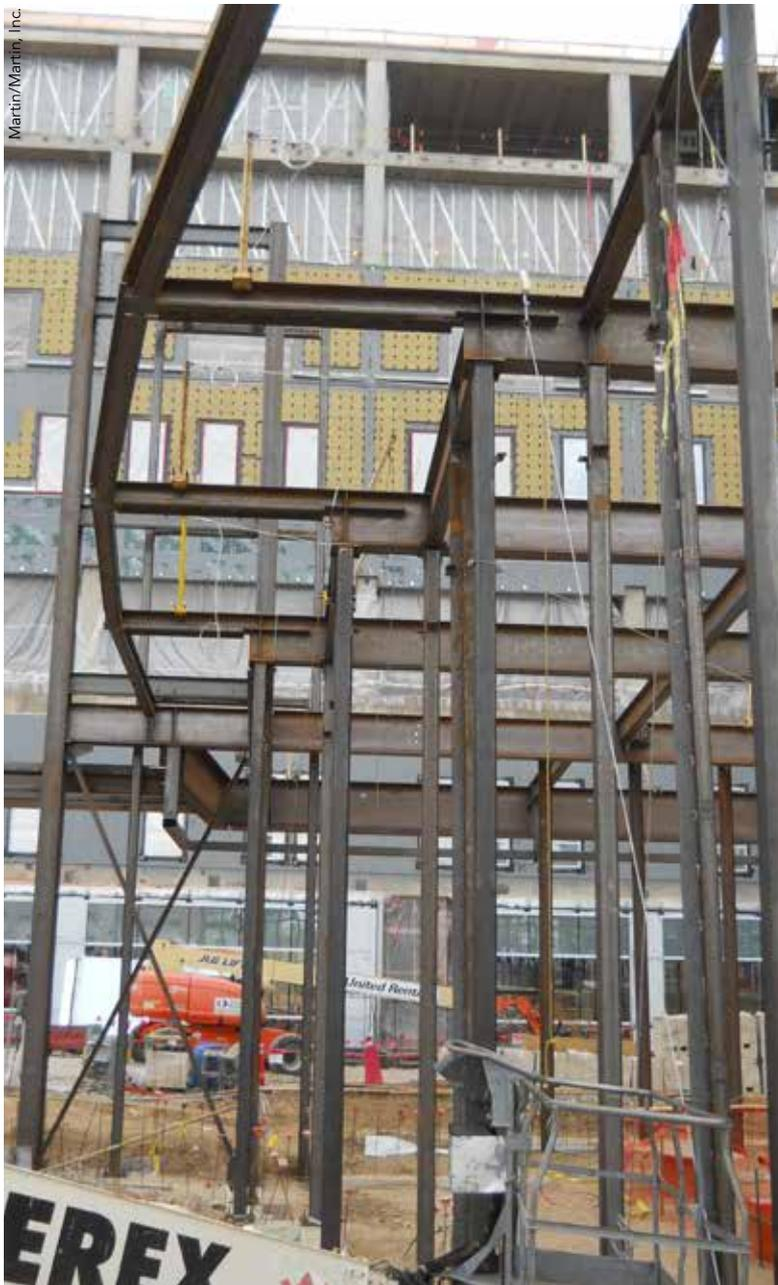
◀ Coped roof beams at the east rake.
