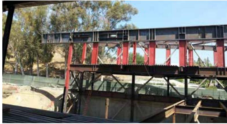
◀ ▲ The natural frequencies of the cantilevered building corners were tuned so that they avoided excitation by the rhythmic forcing frequency of the running motion simulations.
