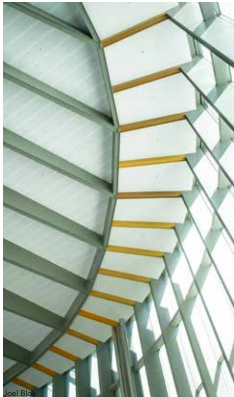
▲ The exposed roof structure lacks the traditional bolted connections seen in long-span trusses or nodes in a space grid.
