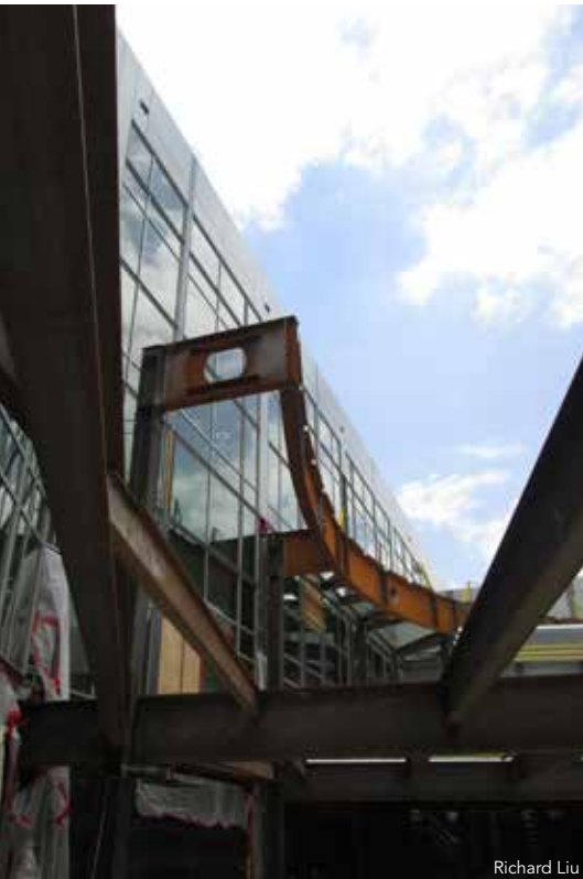
▲ A curved plate girder at the low roof.
