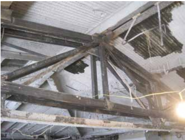
▲ ▼ At some point during the life of the building, three dormers were added to the original sloped roof area. The original structure consisted of cinder-crete slabs, shallow beams and posts down to the floor below, and the main framing bay between building columns was approximately 26 ft wide. Within each of these bays, the original purlins were located 8 ft, 9 in. on center.
