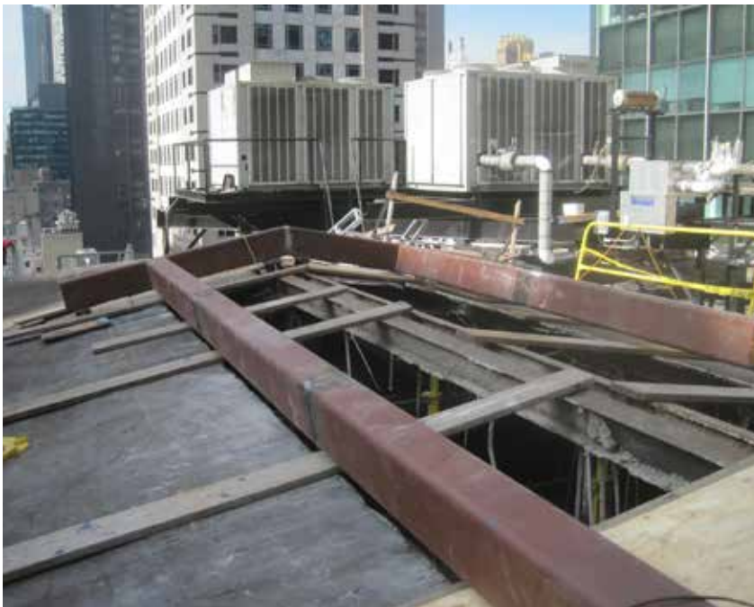
▲ ▼ The structural team decided to support the roof hips with new ridge beams that would span between existing building columns, which were conveniently located at the center of each roof hip's base as well as at the center of each exterior truss.
