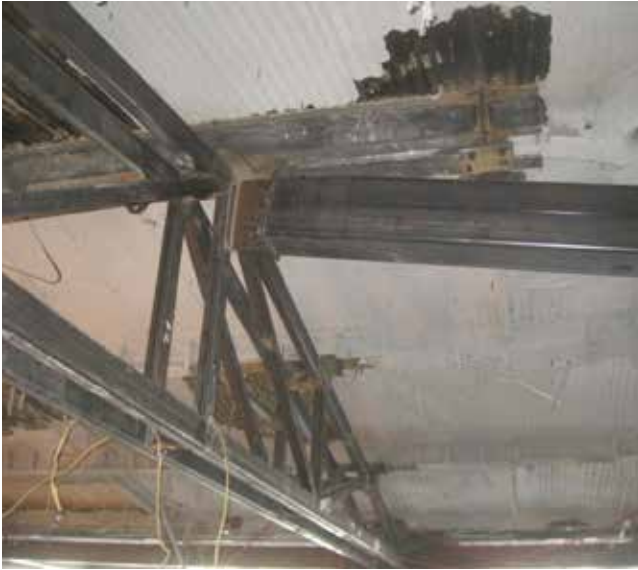
▲ ▼ At some point during the life of the building, three dormers were added to the original sloped roof area. The original structure consisted of cinder-crete slabs, shallow beams and posts down to the floor below, and the main framing bay between building columns was approximately 26 ft wide. Within each of these bays, the original purlins were located 8 ft, 9 in. on center.
