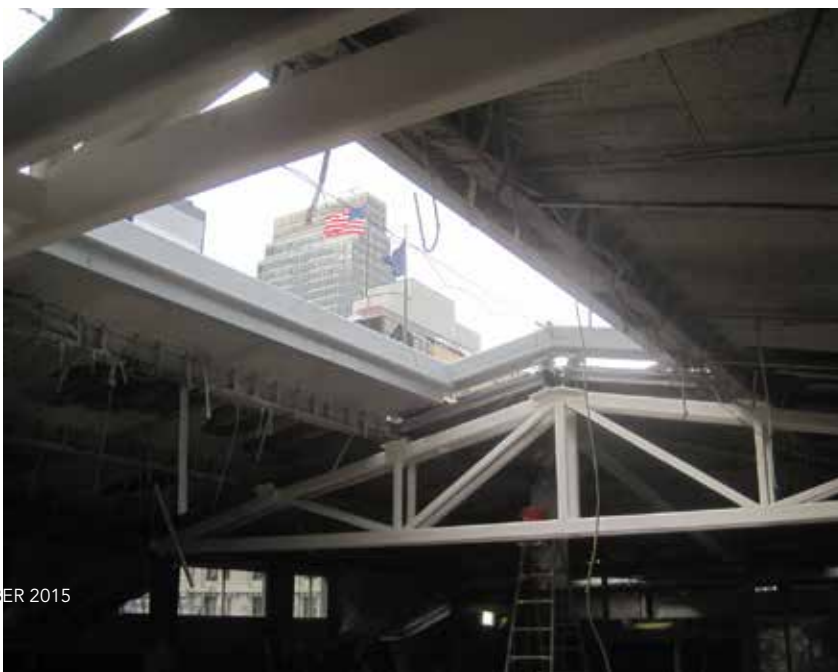
▲ ▼ The structural team decided to support the roof hips with new ridge beams that would span between existing building columns, which were conveniently located at the center of each roof hip's base as well as at the center of each exterior truss.
