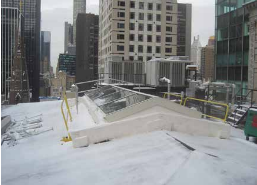
◀ An exterior view of the 25-ft by 8-ft skylight.
