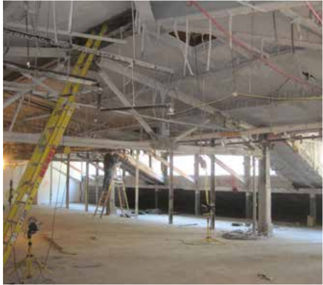
▲ ▼ The skylight also required an additional support structure that would work as an independent framing system and would be located above the roof deck surface. A box frame constructed of HSS12x8 and HSS12x4 members was developed by the engineers and arranged so that the new frame would bear on a total of eight support posts, which were coordinated with the roof purlins below.
