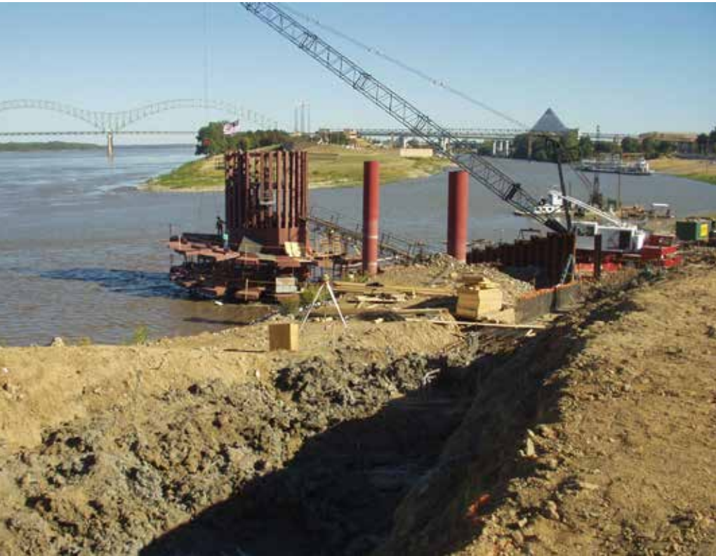
▲ The bridge is supported on two 48-in. HSS columns.
