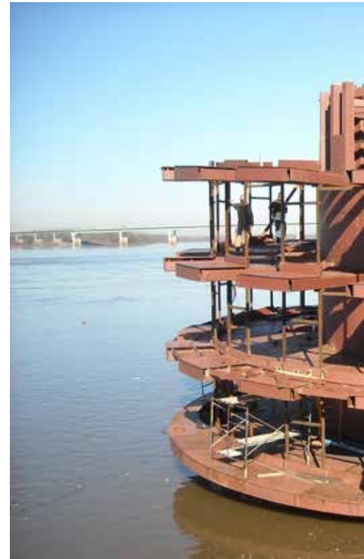
▲ The helical ramp accommodates elevation changes of the floating dock.
