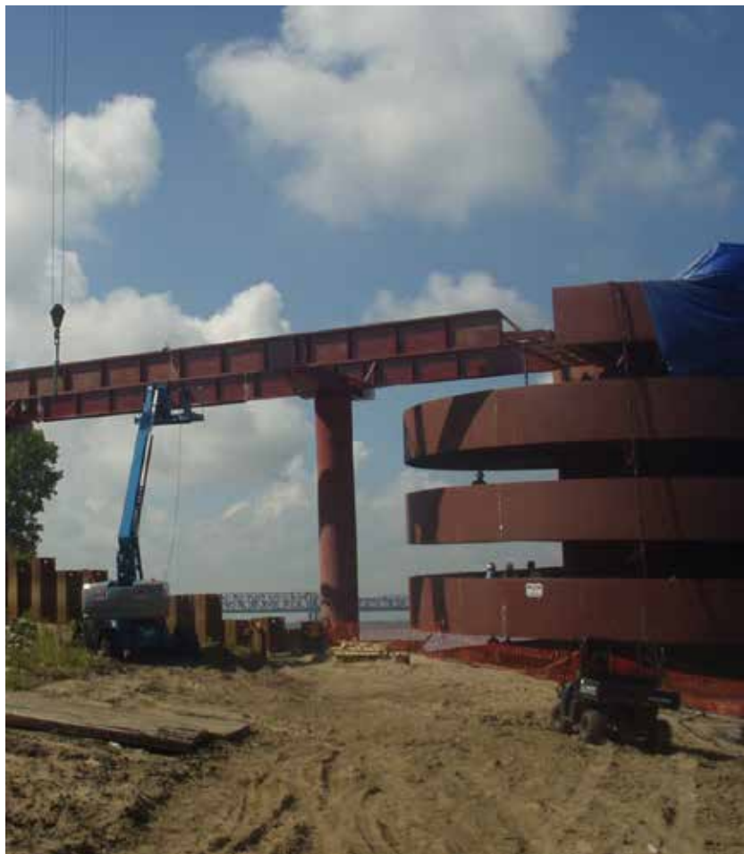
▲ ▼ Framing for the helical ramp consists of 55 HSS12×10×½ columns at the perimeter of a 24-ft-diameter core with ¼-in. steel plate forming the steel cylinder surface.
