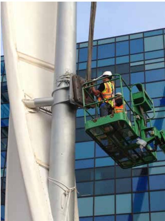
▲ Workers prepare spire connections and templates to be attached to the building support beams.
