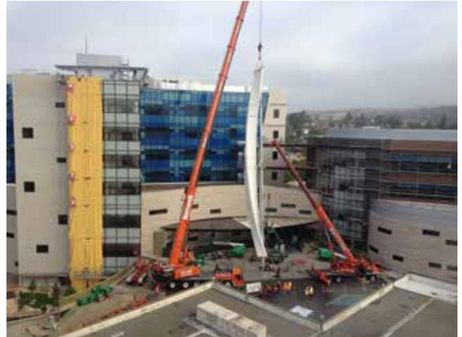
▶ ▼ Interface between the spire and the main building came in the form of double-end plate-type connections with 2½-in. end plates and high-strength bolts.
