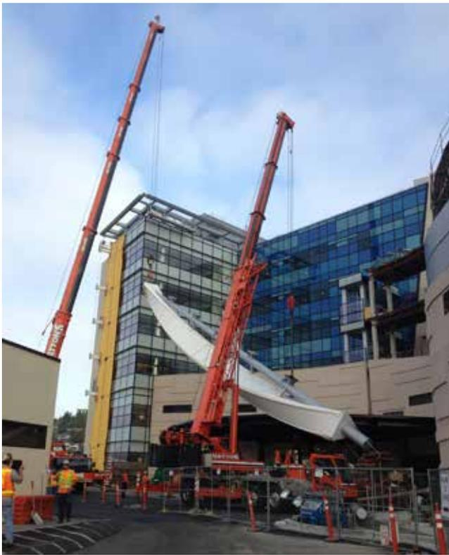
▶ ▼ The spire's shape and length required two cranes for erection in a very tight construction space, given that the building itself was already completed.
