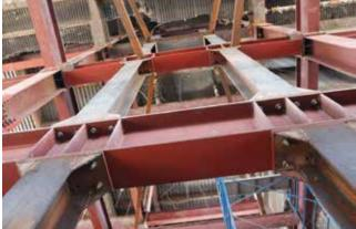
New structural steel. Framing for the main columns was reinforced with HSS lateral supports at each floor.
