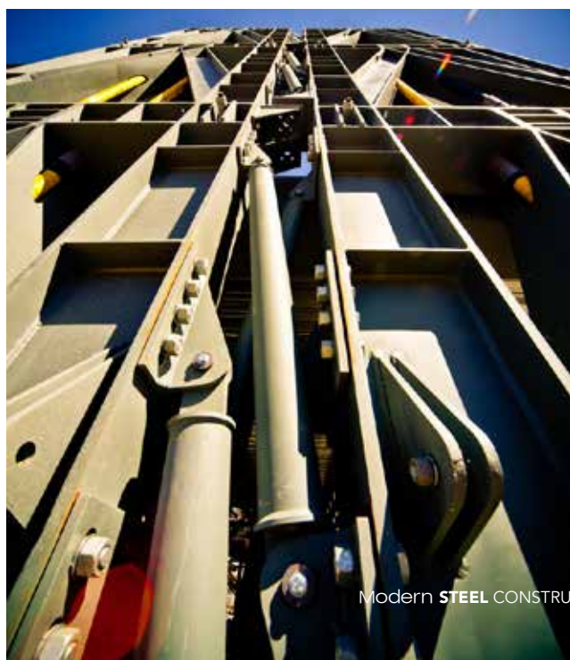
▲▼ The Forte Health Building uses a post-tensioned steel rocking and dissipating system, New Zealand's first application of prefabricated structural seismic system technology.
