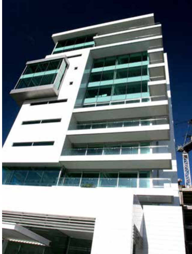
▲ Christchurch's HSBC Tower, which uses an eccentrically braced frame, sustained only minor damage in the 2011 earthquake.
